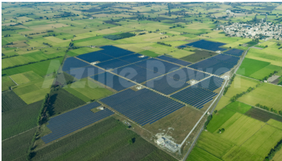
Azure Power Solar Plant (Photo: Business Wire)
